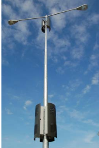
Figure 3: Directional antenna Courtesy of CommScope
