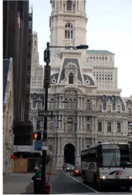
Figure 5: Small-cell equipment can be placed on light poles. Courtesy of Crown Castle
